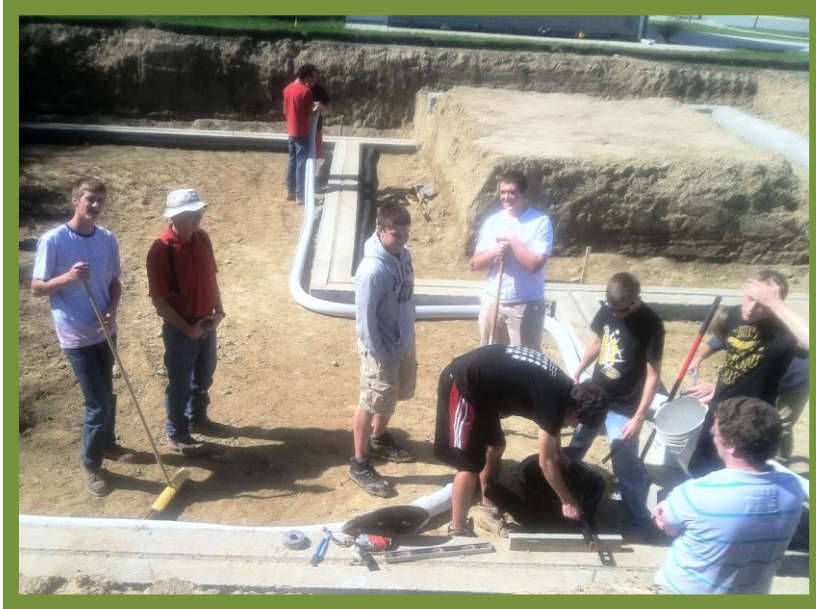
Pictured at left is Mr. Doane's afternoon Construction class working on the drainage tile for the new Building Trades house.
